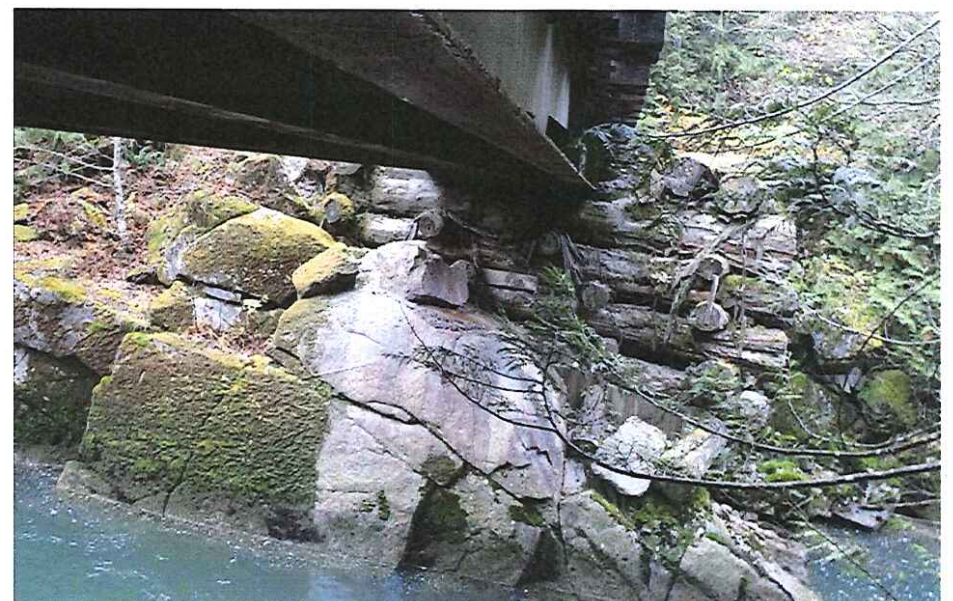
CK2269 Left Abutment
