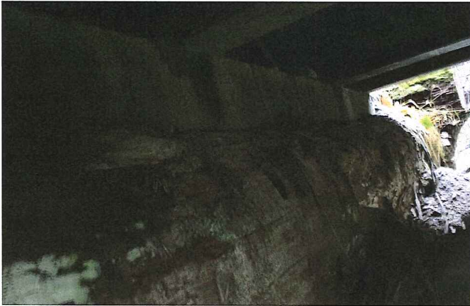
CK2269 Right Abutment
