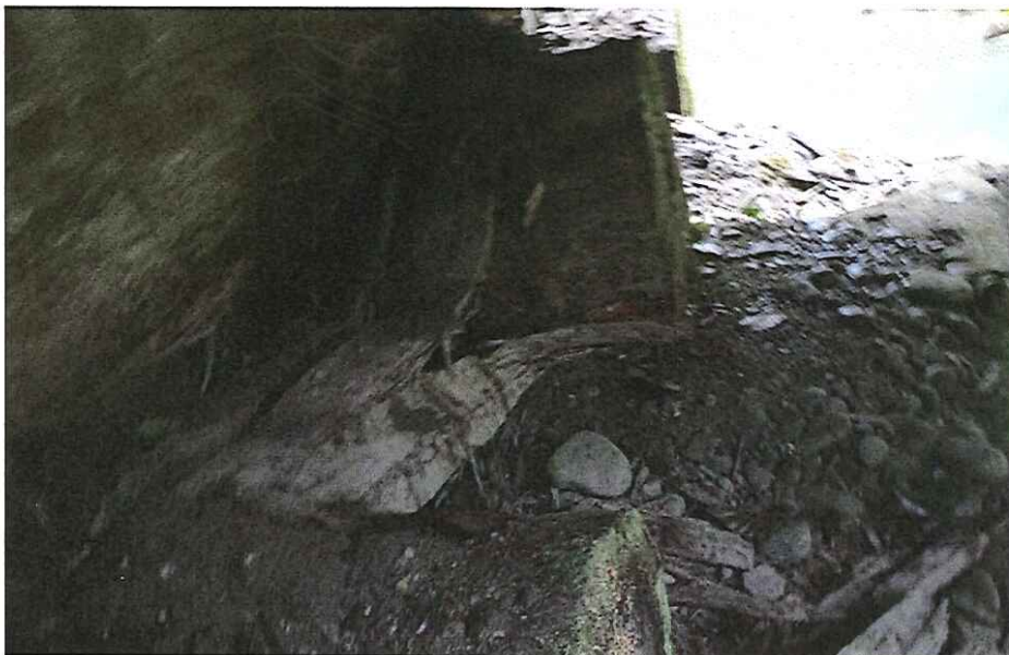
CK2269 Right Abutment 2
